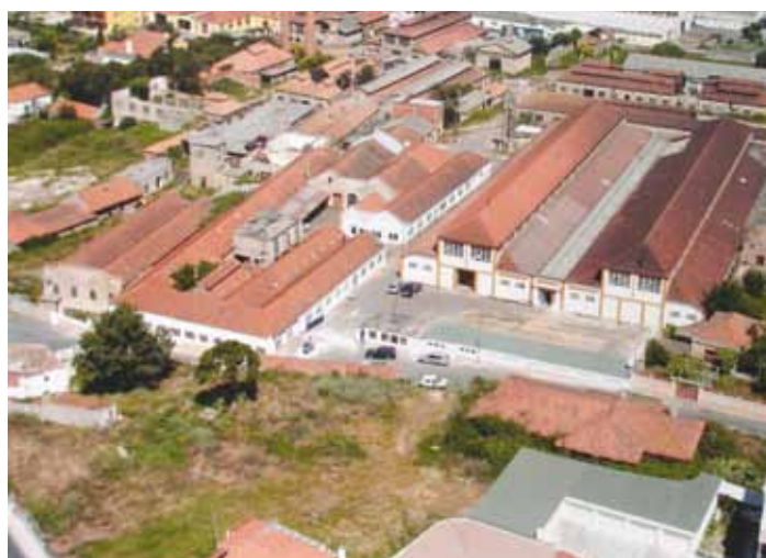
Aerial Plant View
